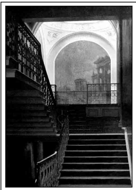
18 th century staircase with wrought-iron balustrade.
